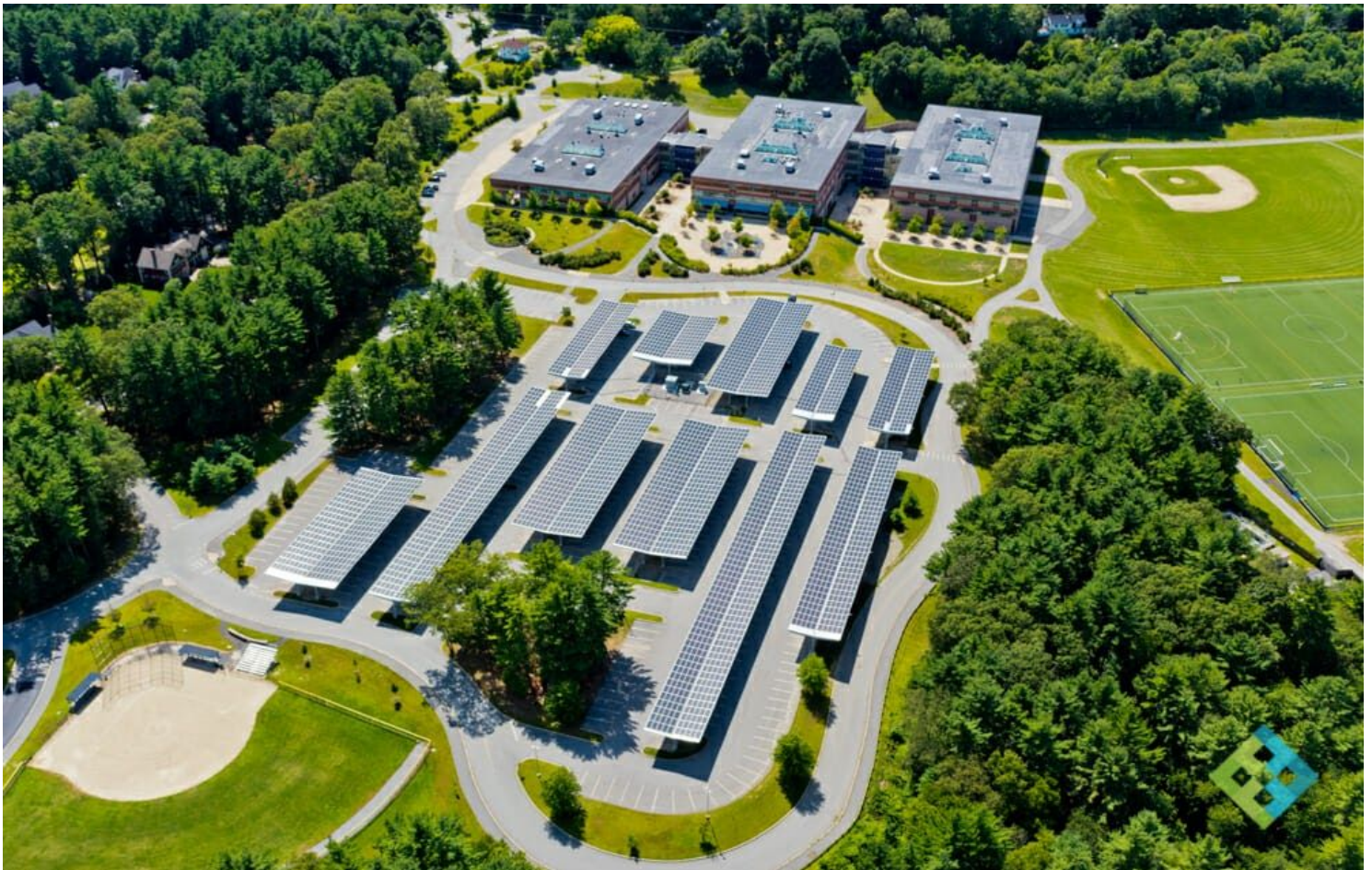
L-S SITS ON 93 ACRES OF PROPERTY that B&G is responsible for maintaining. Photo courtesy of ForeFront Power.
